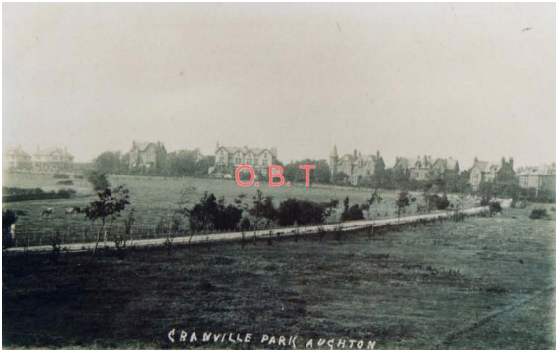
Photograph showing first phase of development in Granville Park
